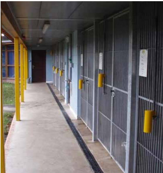
Protected external runs (showing drainage)
